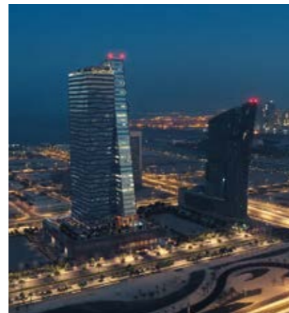
Lusail Office Tower, Qatar
