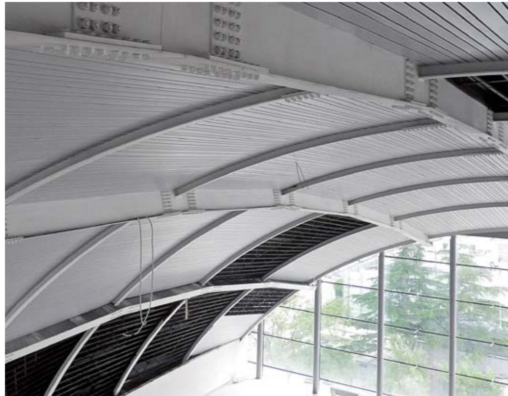
Baffle linear strips system 40/150 ral 1035 Forest Office City · Debrecen, Hungary
